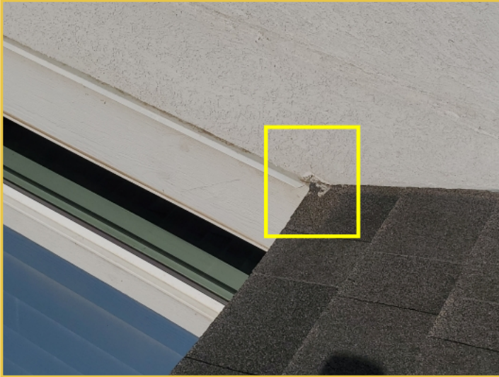
Short Kickout Flashing
