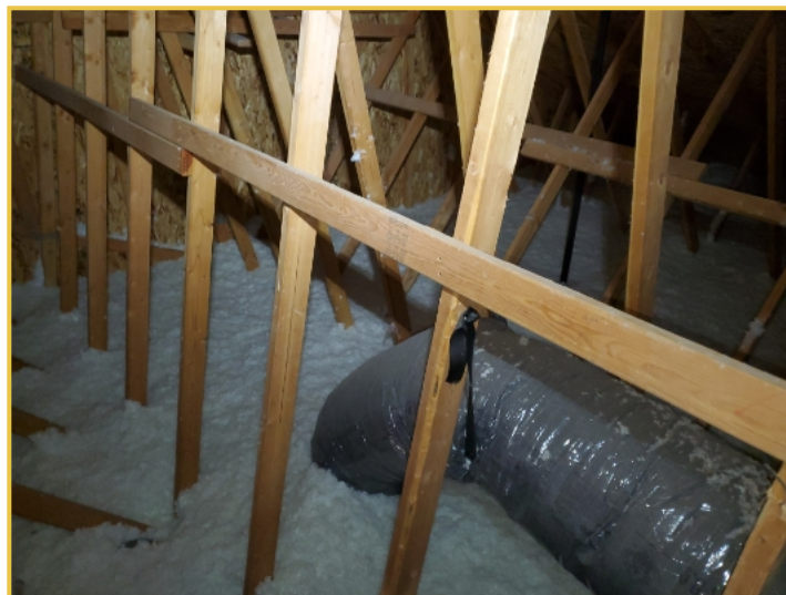
Attic With Fiberglass Insulation
