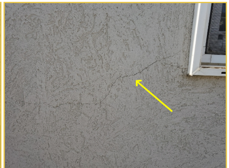
Cracked Stucco Siding at the Window
