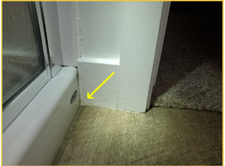
Evidence of Past Leaking at the Basement Bathroom Baseboards That Was Dry
