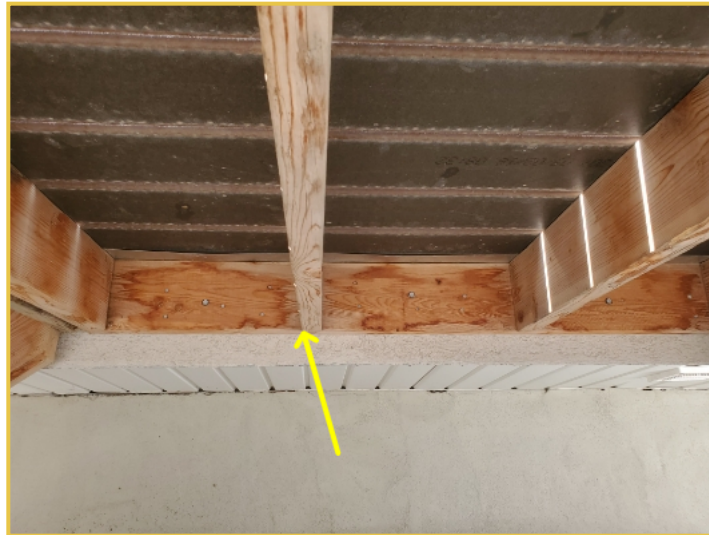
Missing Fasteners
