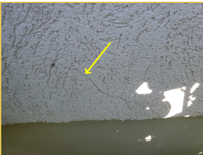
Cracked Stucco Siding
