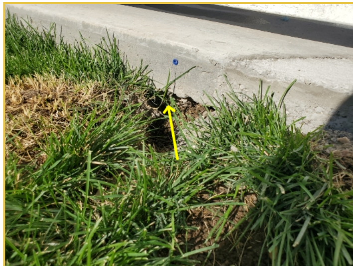
Void Under The Rear Concrete
