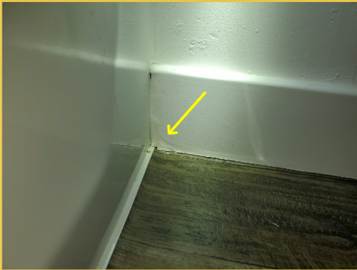
Evidence of Past Leaking at the 2nd Floor Full Bathroom Baseboards That Was Dry
